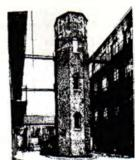
Entry to the floors was made by stairs accommodated in towers (one at each end of the courtyard), lit by narrow windows. On every floor, the tower is connected to the building by an open iron, footbridge. A short balcony along the facade gave access to the different areas.
